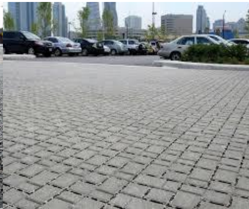
Fig 6 Interlocking concrete (Source: 3riverswetweather.org)
