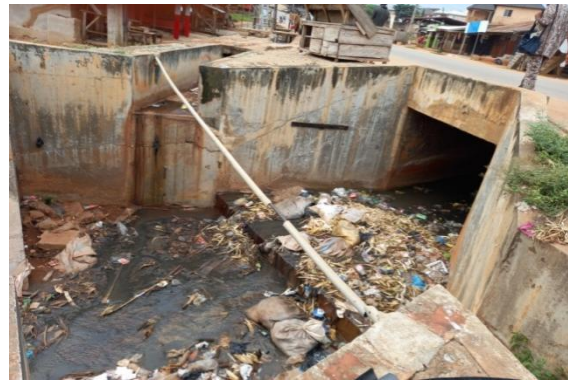
Fig 4c: Submerge Building in flood
