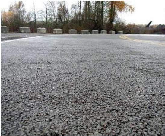
Fig 5: Permeable Concrete (Source: roohome.com)
