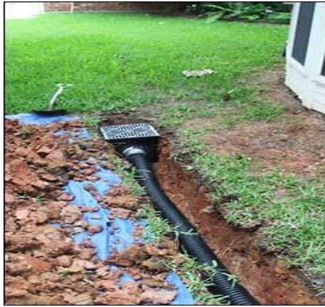
Fig 2. Buried Pipe Drain
