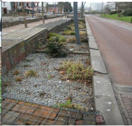
Fig 3. Downspout and Gutter systems (Source:
