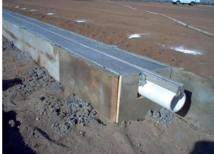
Fig 3. A Slot Drain System (Source: sportsedge.com)
